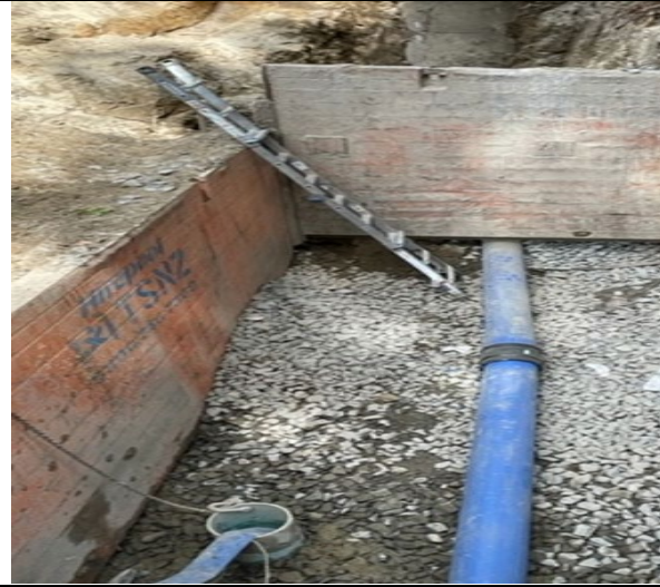
Photo 4: Repaired Pipe at Primary School
