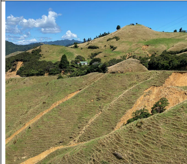
Photo 11: Mangatōa Road Landslips
