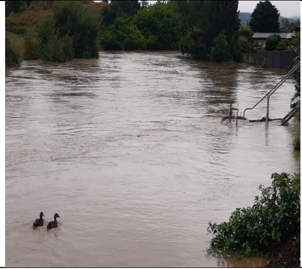
Photo : Te Kumi WWPS during the flood
